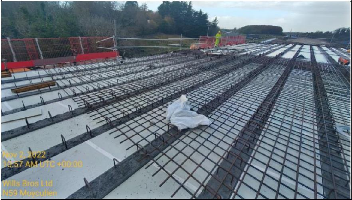
Installation of Steel Reinforcement for ST07 Lough Kip River Bridge Deck Pour
