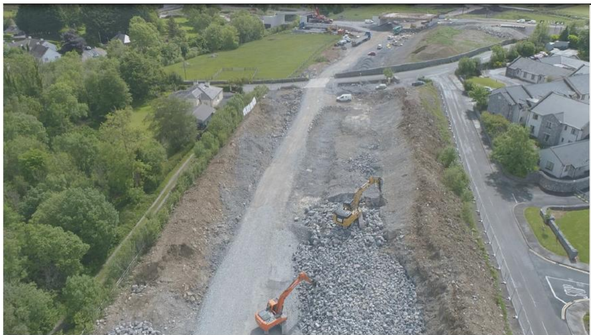
Rock Breaking at Cut 02 Adjacent Knockferry Road
