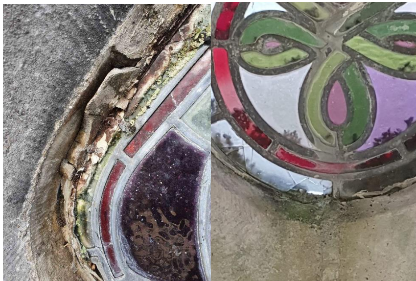
Gloine scoilte, luaidhe na fuinneoige lofa, alga ag fás mar gheall ar uisce ag teacht isteach
