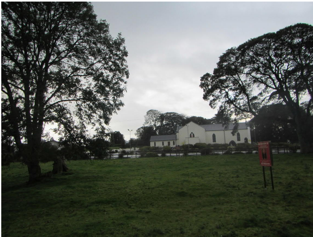
Photograph 14.22 The Protected Structure St. Bernard's Church (No. 83).
