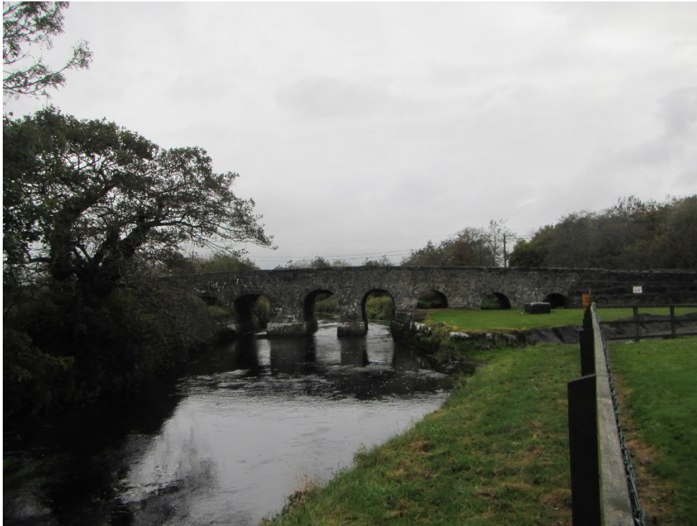
Photograph 14.19 The Protected Structure Liss Bridge (No. 3925).
