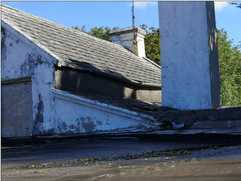
Plate 4. Roofs of Building BLD02 offering some potential roost locations
