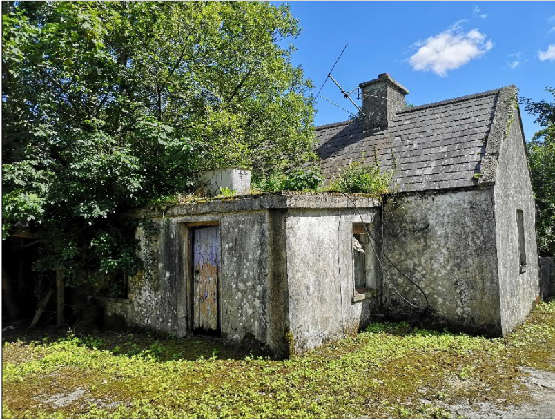
Plate 5. Rear view of Building BLD03. Classified as having 'Moderate' bat roost potential.
