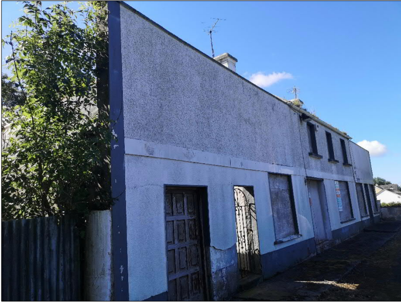
Plate 3. Front view of Building BLD02
