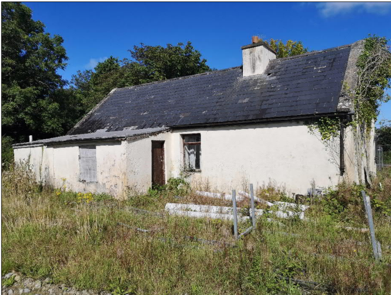
Plate 2. Rear view of Building BLD01.
